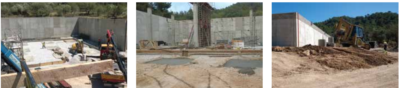
Fig 2: Progress photos taken during construction of the reservoir (photos courtesy of CAT)
